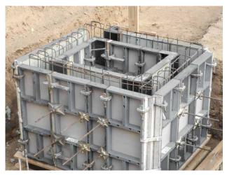
By using inside and outside corners as well as continuously adjustable hinged corners, it is possible to form all angles between 0° and 180°.
